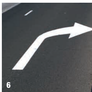
1 Cold Applied Plastic (sprayed). 2 Anti-skid treatment. 3 Raised pavement markers. 4 Raised pavement markers. 5 Cold Applied Plastic (roll on). 6 Thermo-plastic. 7 Thermo-plastic. 8 Oil-based paint.
