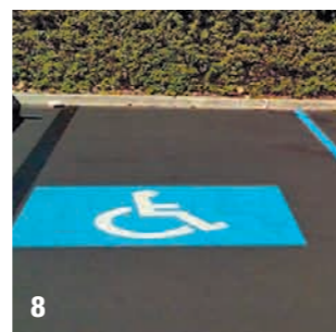
1 Cold Applied Plastic (sprayed). 2 Anti-skid treatment. 3 Raised pavement markers. 4 Raised pavement markers. 5 Cold Applied Plastic (roll on). 6 Thermo-plastic. 7 Thermo-plastic. 8 Oil-based paint.
