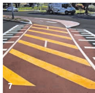
1 Cold Applied Plastic (sprayed). 2 Anti-skid treatment. 3 Raised pavement markers. 4 Raised pavement markers. 5 Cold Applied Plastic (roll on). 6 Thermo-plastic. 7 Thermo-plastic. 8 Oil-based paint.
